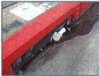
Figure 3.9 Typical opening cover after rain event less than 0.25in (3/29/06)
