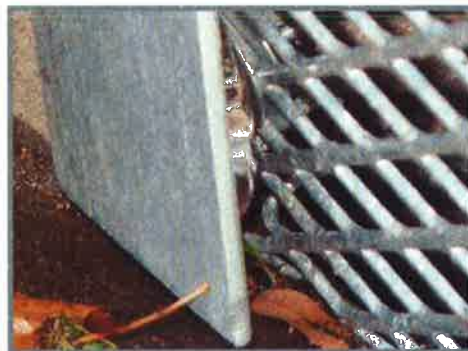
Figure 1.5 Typical Opening Screen Cover Magnet Locking Mechanism
